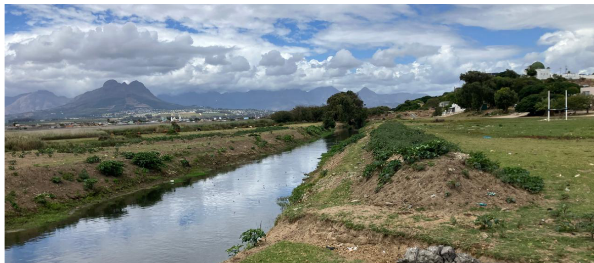
Photograph 5.1. Inappropriate and possibly unauthorised construction of a flood protection berm along the edge of the Eerste River to prevent flooding of the adjacent sports field puts increasing pressure of erosion and flooding on wetlands downstream.
