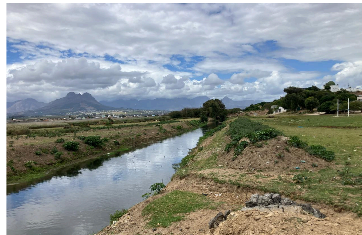
Photograph 4.2 Berm created along the edge of the Eerste River, to protect adjacent sports field and higher-lying Residences from flooding. The berm is however likely to increase flood impacts on important downstream wetlands, and its (unauthorised) construction highlights the problem of allowing settlements in riverine floodplains and the importance of understanding that so-called benign floodplain uses such as sports fields need to take cognisance of the fact that floodplains are by definition periodically flooded.
